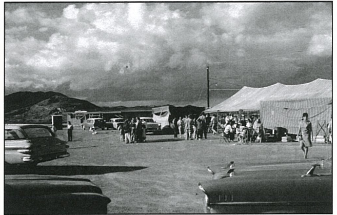
CONGREGATION MET IN TENT BEFORE CONSTRUCTION OF CHURCH
