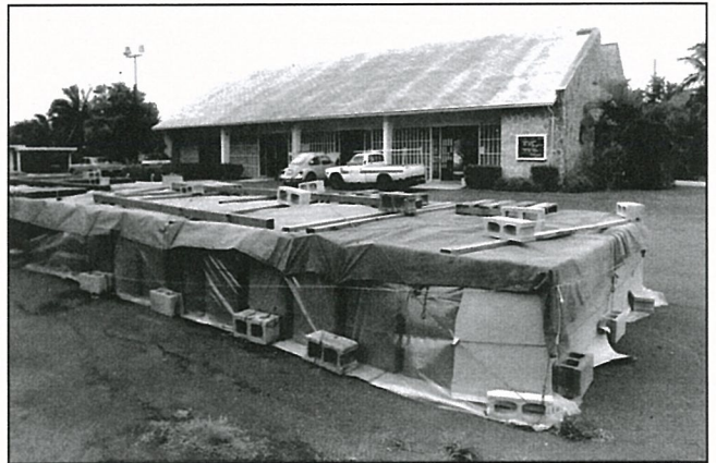
CHURCH UNDER CONSTRUCTION
