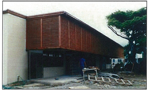
CONSTRUCTION OF PARISH HALL
